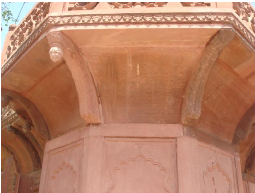
Taj Mahal, Agra: before and after conservation of Fatehpuri mosque, broken and decayed stones,
