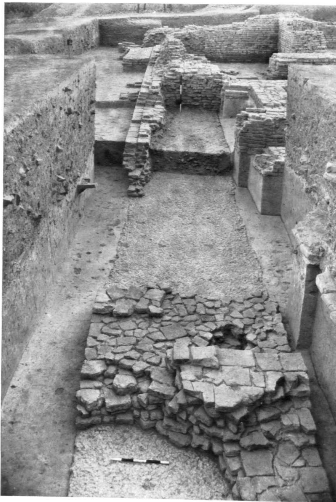
Bhitari : damaged eastern wall. See p. 47
