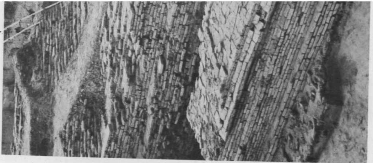
69. Ballalधिpi brick-built compound wall.
