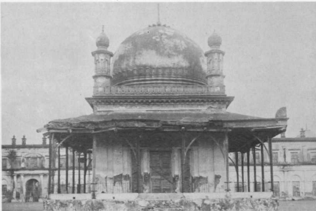
115 Murshidabad, Hazar-duari Palace before conservation of Madina Mosque.
